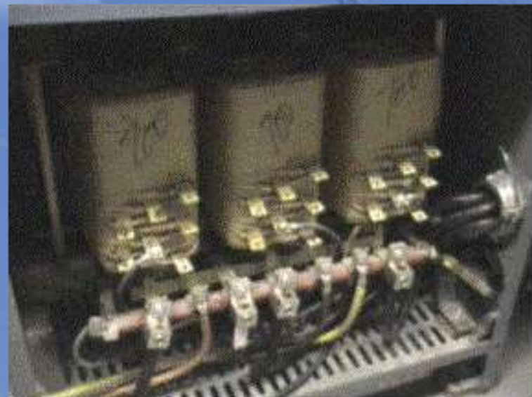
Above thermal and daylight images show uneven heating in the windings of a three phase step-down transformer, most likely due to harmonics.
